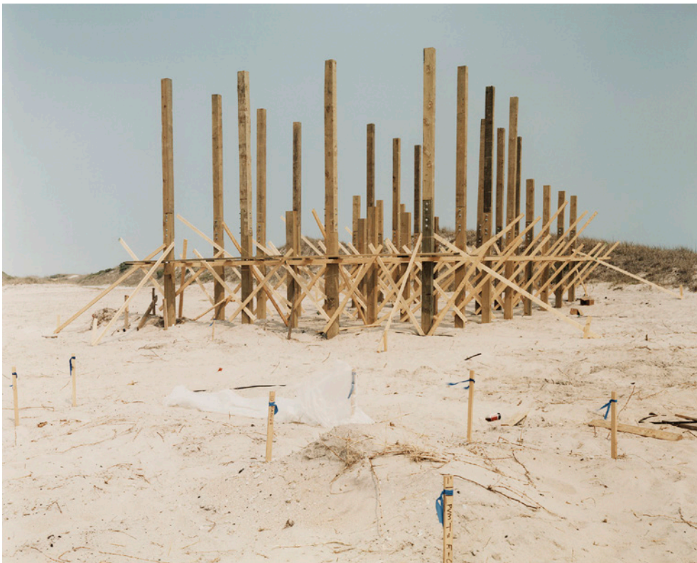
Peter Goin. Public beach access structure under construction north of Surf City, North Carolina, on the Outer Banks , 1992, digital pigment print. © Peter Goin, Courtesy of the artist.
